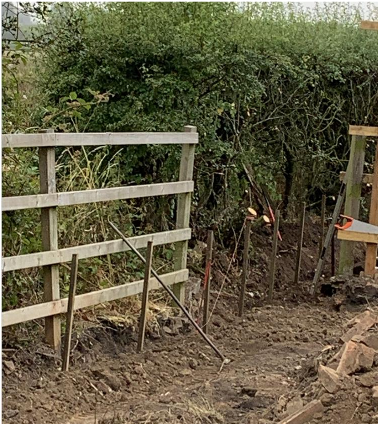
Photo to show depth of hedge removal
