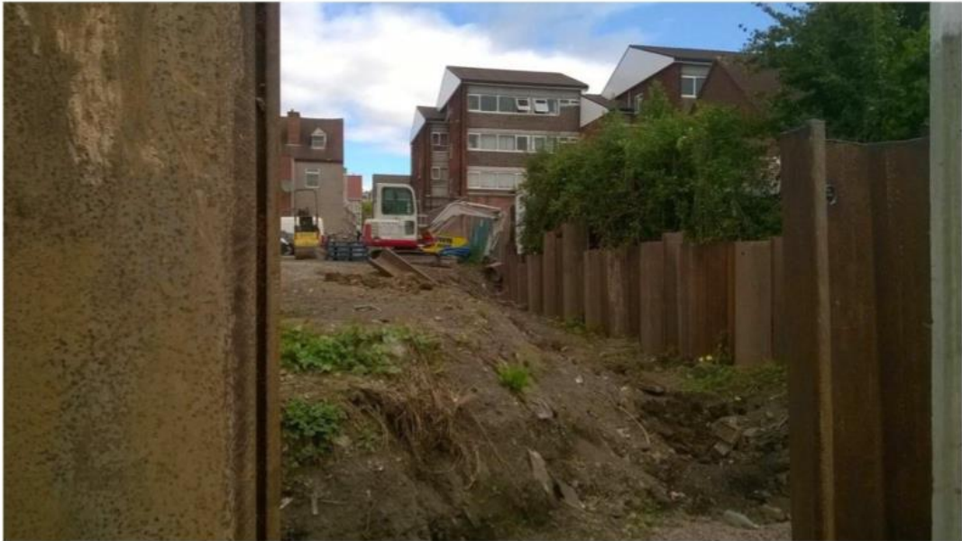
Photograph looking north towards Coleshill Road – Chancery Lane on right during development
