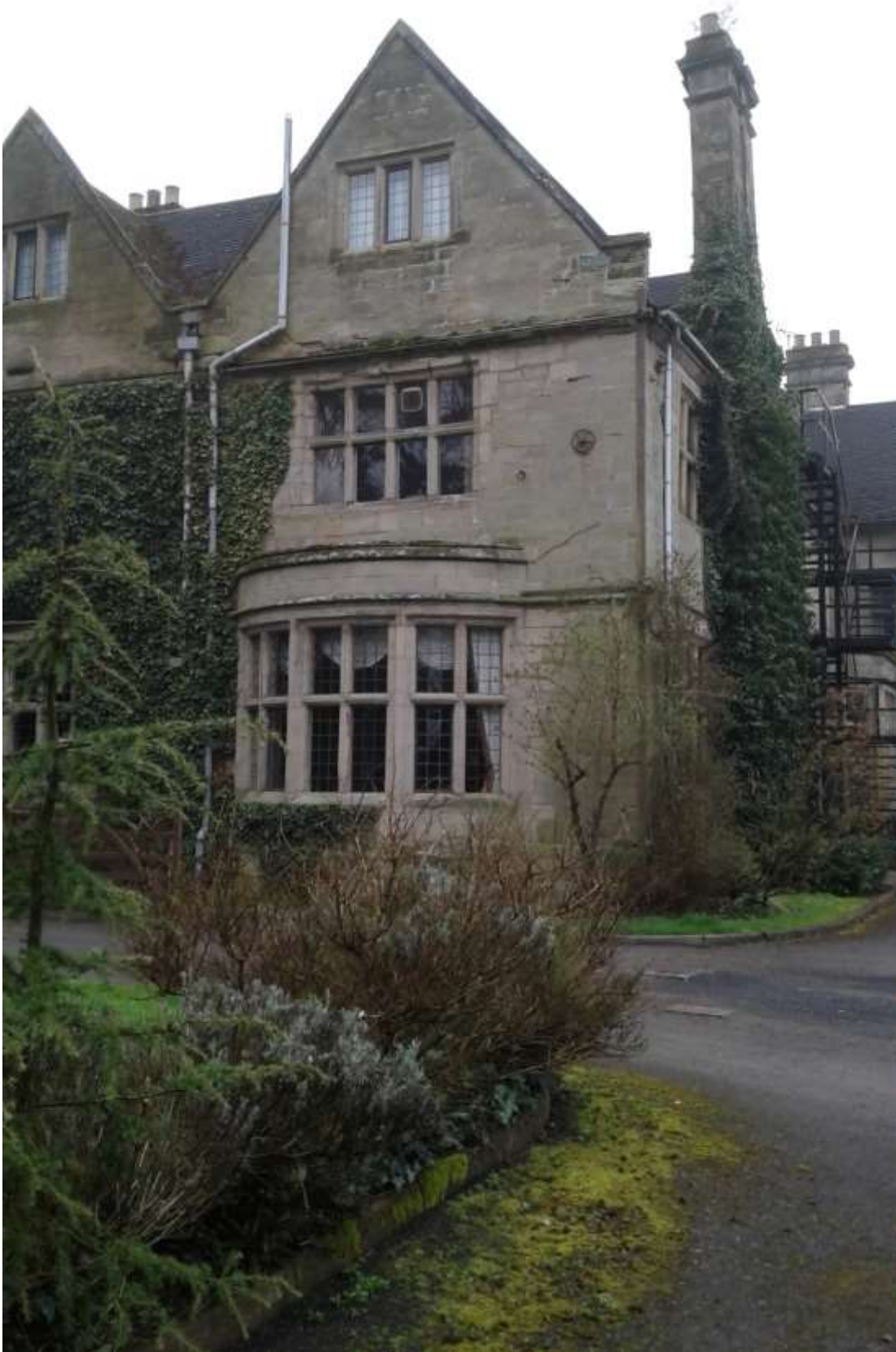
Photograph of corner of building (East) closest to the marquee
