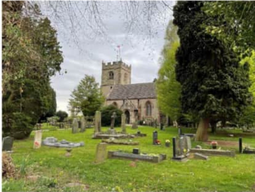
VIEW LOOKING NORTH-WEST TOWARDS GRADE II* LISTED CHURCH OF ST GILES
