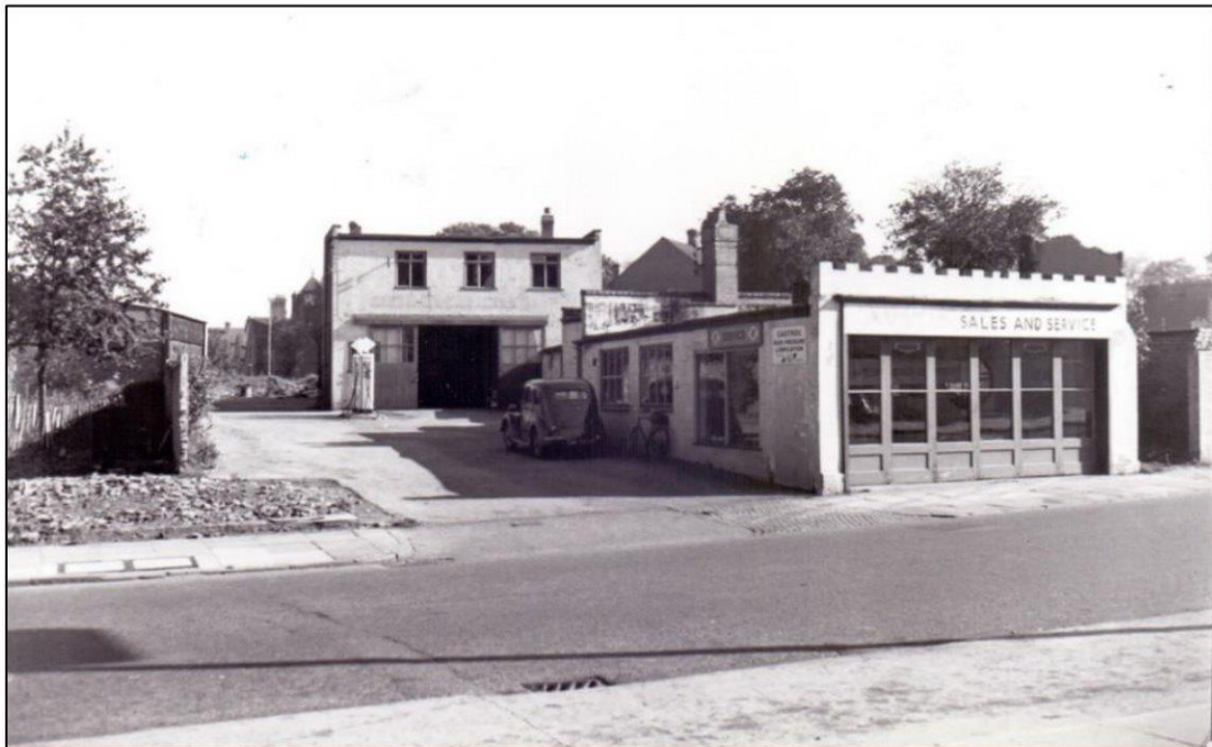
The site of the new library in Church Street before development. The former car showroom garage fronted Church Street and the workshop at the rear was on the side of the library. The garage building, was used by the library builders G.E. & W. Wincott of Coton Road, Nuneaton for storage of materials once construction work on the new library started. The workshop we
