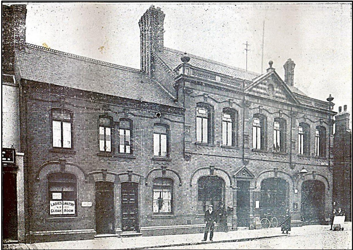
The old fire station with council offices above and ladies lavatory, the only WC for females available in town at the time. The fire station was converted into the library in 1934, but would prove inadequate accommodation by the 1950's. (NLHG Archives)
