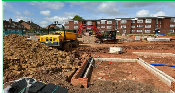
New build start at Byfield Street, Bar Pool
