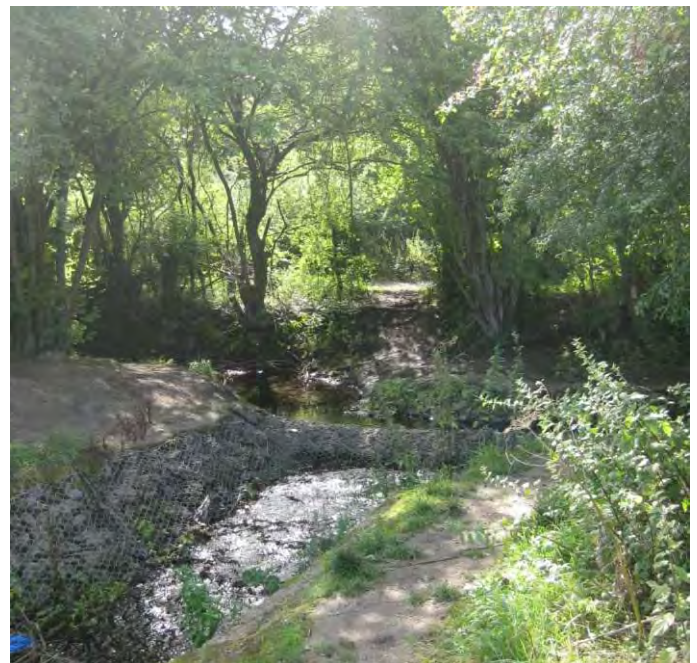
Bank Strengthening works carried out along the wooded river valley
