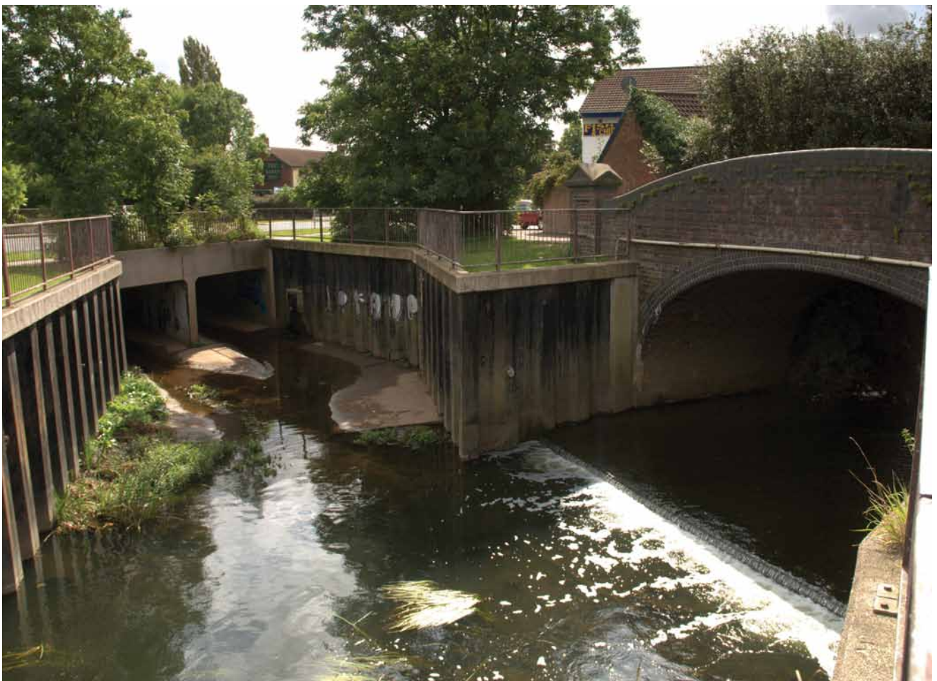
↑ River Anker culvert, Nuneaton
