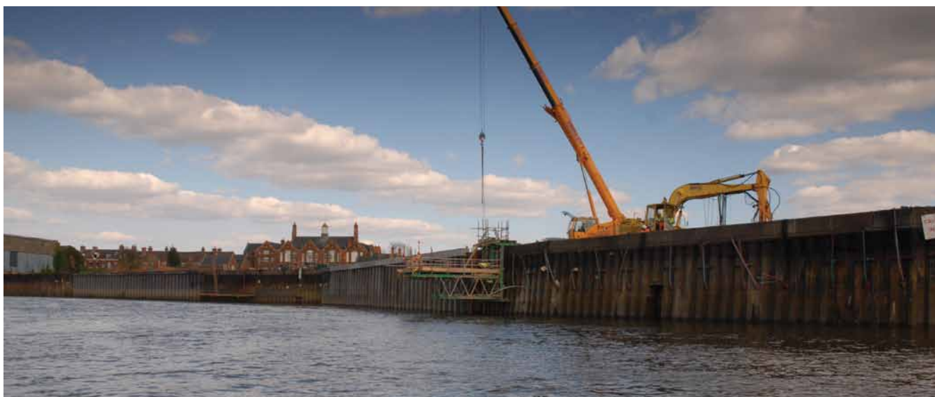
↑ Flood defences, Gainsborough
