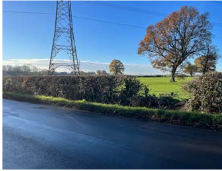
Electricity pylons and trees within the site
