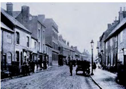
Abbey Street (now demolished)
