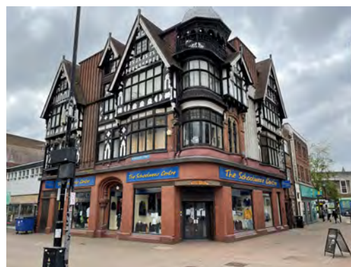
Former Gate Hotel, Nuneaton today
