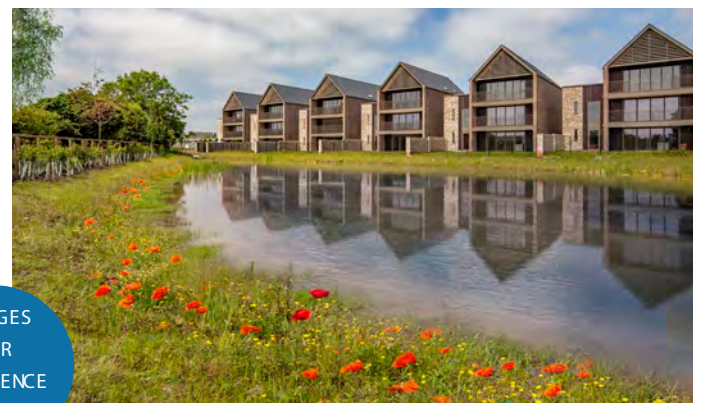
Example of water storage solution at Ninewells, Cambridge (Hill Group)
