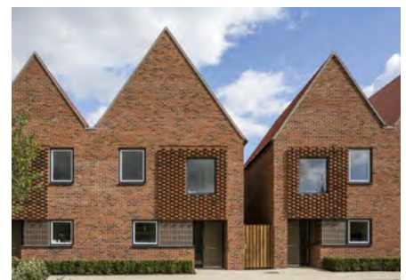
Suitable access provided between semi-detached homes at Horstead Park providing rear access for bin and bike storage.
