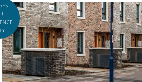
Meters and utilities integrated alongside parking areas at Marmalade Lane, Cambridge
