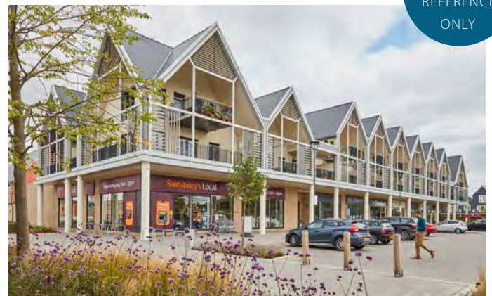
Beaulieu local centre (Countryside Properties)
