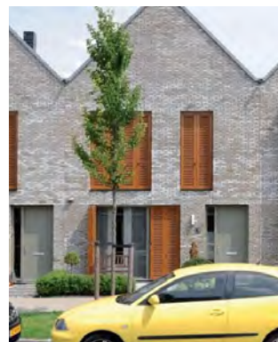
Deep window reveals enable external shutters to aid with solar shading
