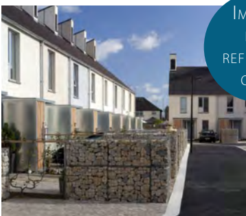
Storage for bins and bikes is sensitively integrated within front defensible space at The Triangle, Swindon
