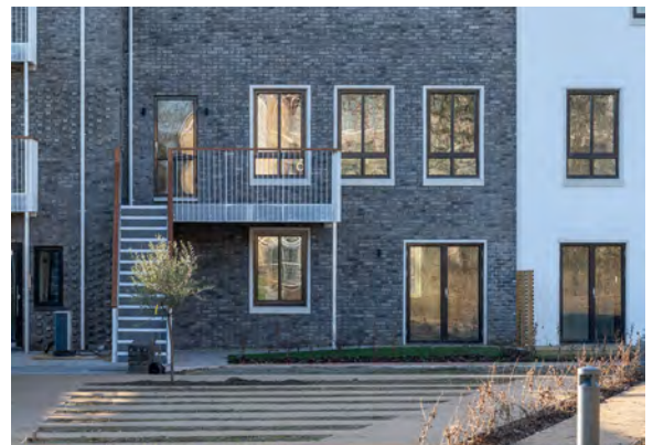
Walk-up apartments at Marmalade Lane
