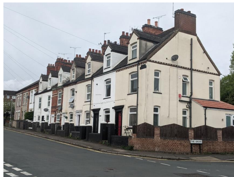
Figure 48: Chapel Street, Original Brickwork in the Middle Property.
