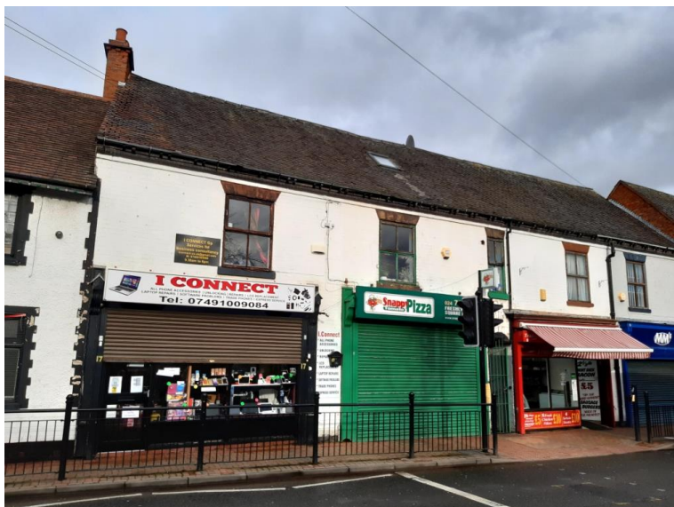
Figure 29: Shop Fronts, Mill Street
