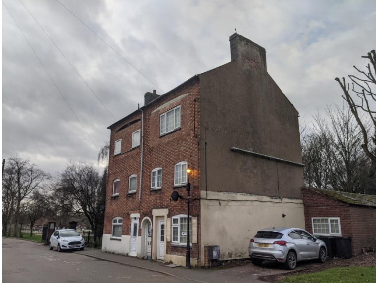
Figure 5: Three Storey Top Shop off Rye Piece Ringway
