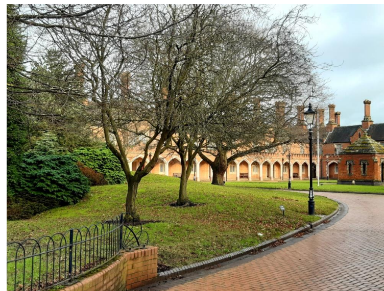
Figure 30: Bedworth Almshouses, All Saints Square
