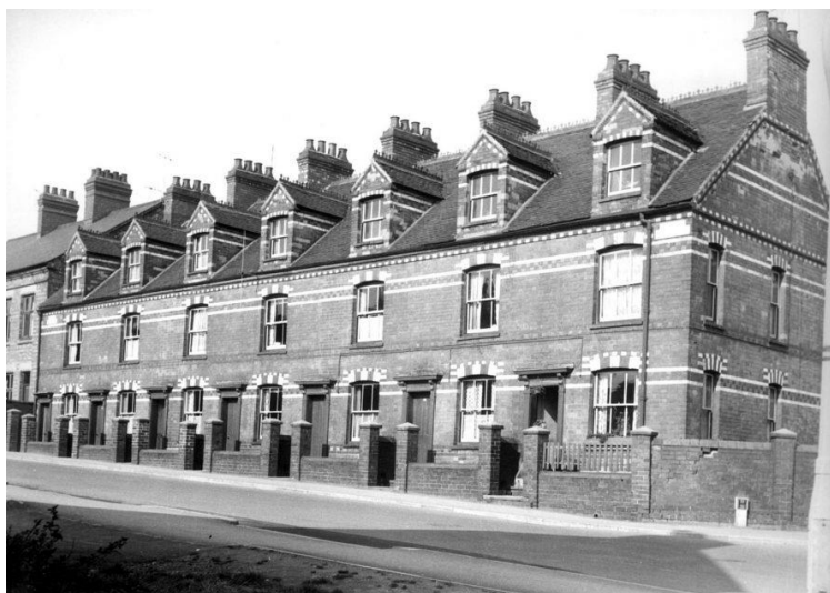
Figure 47: Terraced houses Chapel Street, 1920s 31
