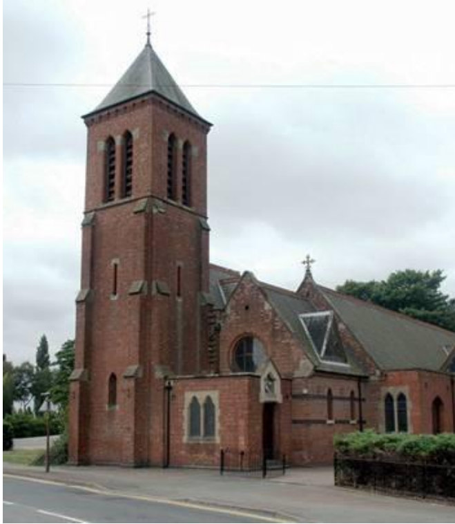
Figure 14: St Francis RC Church, Rye Piece
