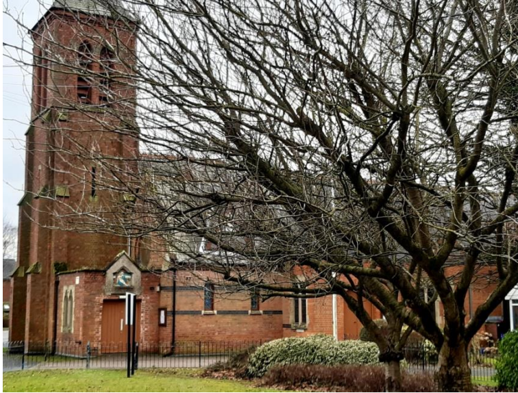
Figure 57: St Francis RC Church
