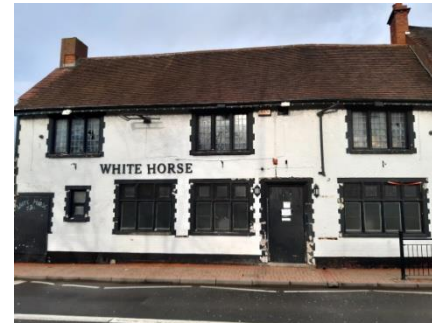
19 Mill Street, White Horse Public House
