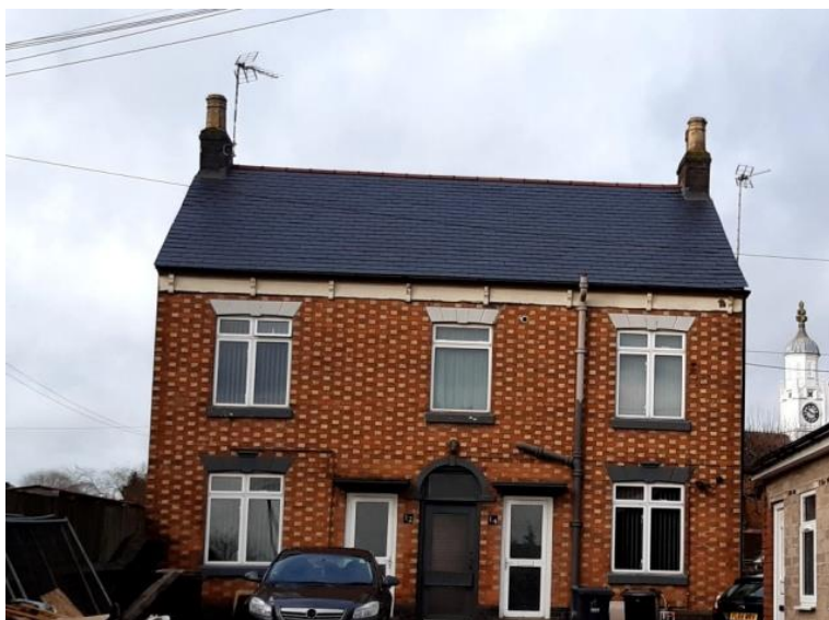
Figure 31: Distinctive Brickwork, Croxhall Street
