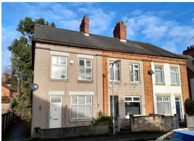
Figure 61: Satellite Dishes, Exposed Wires, Cladding
