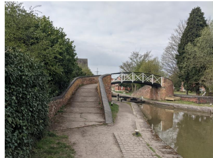
Figure 13: View 3 Roving Bridge Over the Oxford Canal
