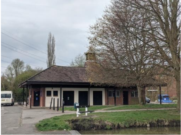
Figure 25: Central Services Building
