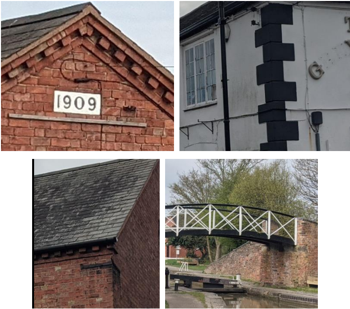
Figure 8: Decorative Details and Signage
