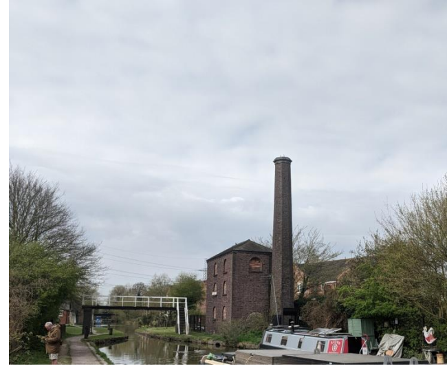
Figure 16: Northern Bank of Coventry Canal
