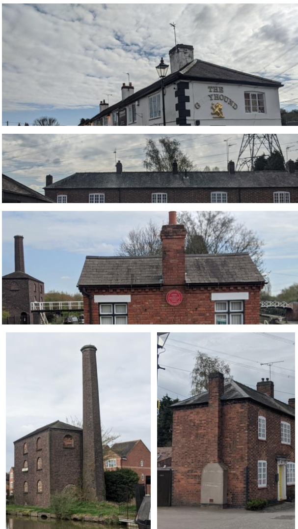
Figure 9: Roofs and Chimneys
