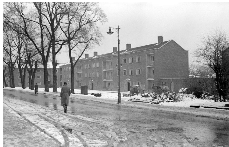
Figure 62: Dempster Court flats seen from the corner of Vicarage Road. 1952 36
