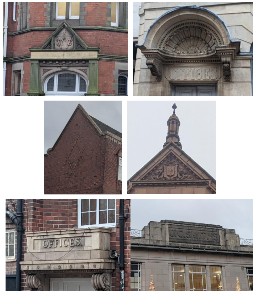
Figure 27: Decorative Details and Signage
