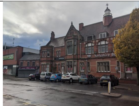
Coton Road former Council Office Positive
