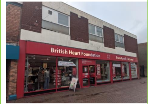
6 to 14 Stratford Street Neutral
