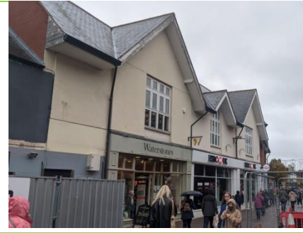
Queens Road (Waterstones)
