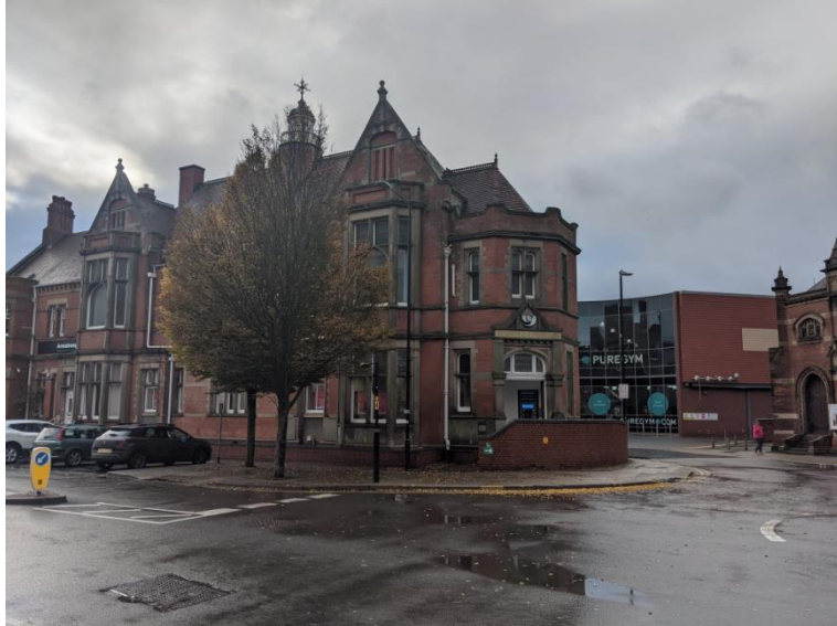
Figure 53: Former Nuneaton Police Station and Magistrates Court, Coton Road. 2021
