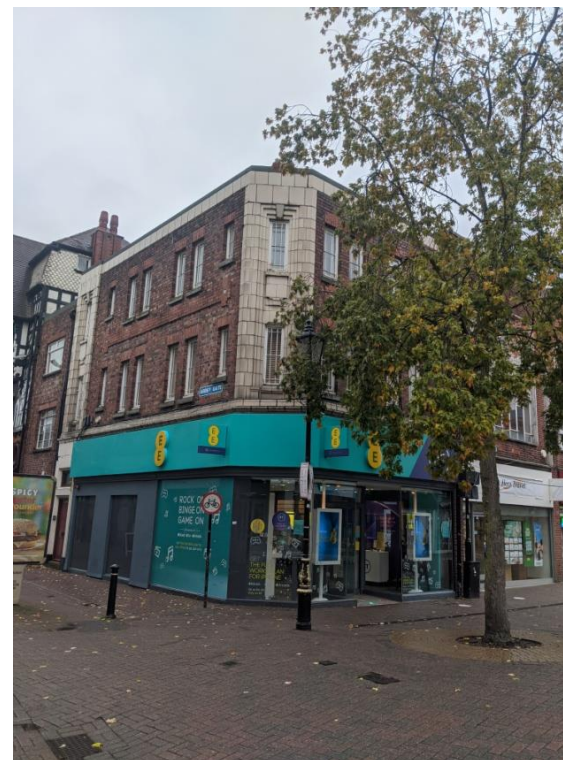
Figure 24: National companies can bring welcome visitors to the conservation area. However, the signage does not always integrate with the architectural building style.
