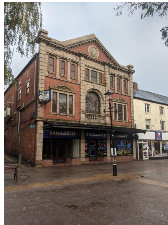
Figure 48: 121-122 Abbey Street Former Scala Cinema
