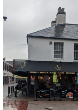
Corner of Queens Road/Stratford Street
