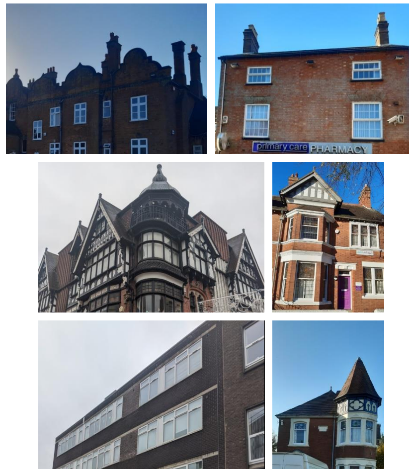
Figure 28: Roofs in the Conservation Area
