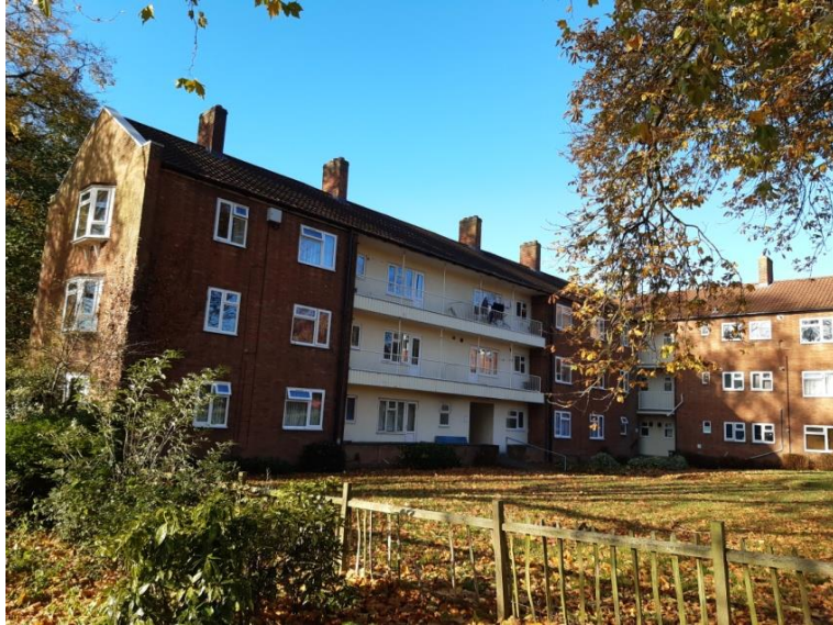
Figure 63: Dempster Court, Church Street
