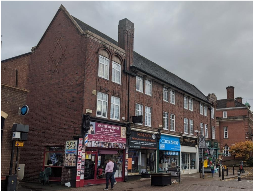
Figure 25: George Elliot Buildings, Coventry Street, feature some original shop frontages.
