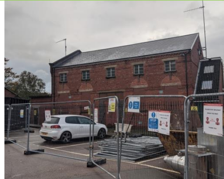
Sub Station rear of Town Hall Neutral
