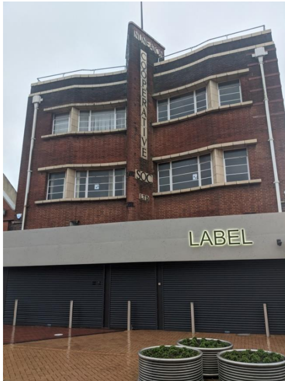
Figure 40: 23a Queens Road (Former Co-op Building)
