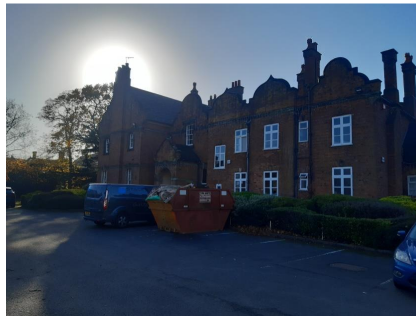
Figure 67: The Old Vicarage, Vicarage Street
