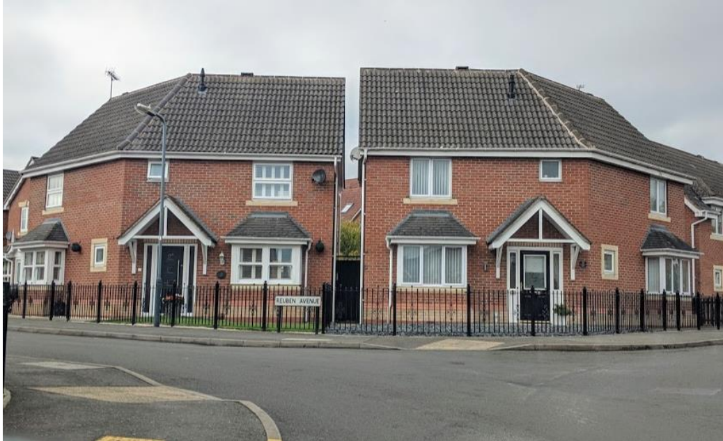
Figure 9: Development at Chapel End, Nuneaton has created homes following the contour of the road
