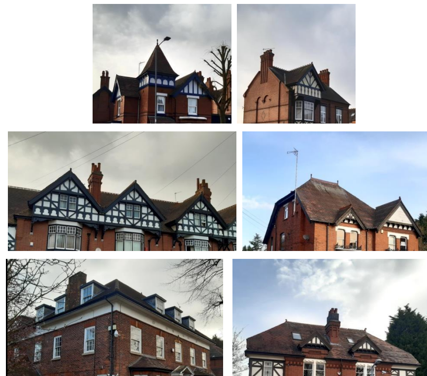
Figure 37: Roofs in the Conservation Area
