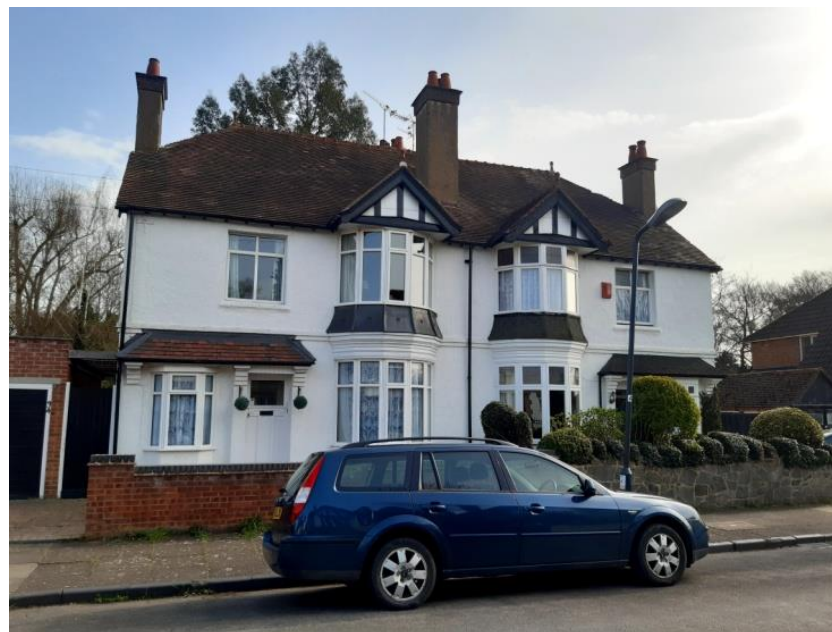
Figure 28: 34-36 Manor Park Road c. 1920 by architect Ernest Shepherd for George Cooper
