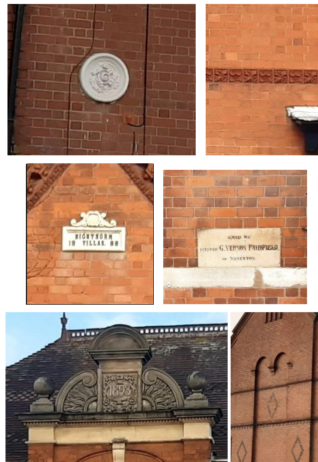
Figure 36: Decorative Details and Signage
