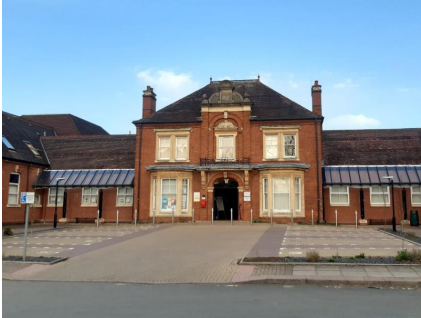
Figure 12: The former Cottage Hospital 1893 by F J Yates
