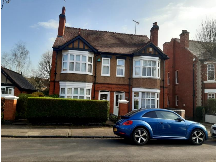
Figure 24: 6-8 Manor Park Road 1909. Designed by H Mayo & Son
