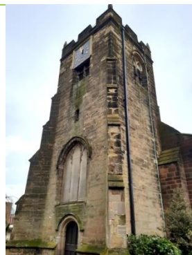
All Saints Church Grade II* Listed Building - Positive
