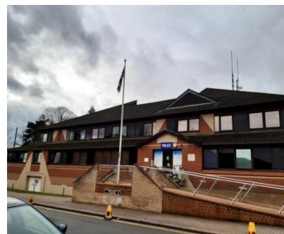
Police Station, High Street Neutral
