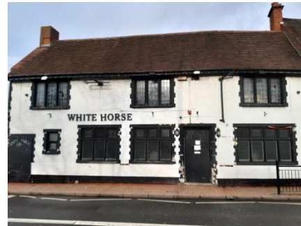
19 Mill Street, White Horse Public House
