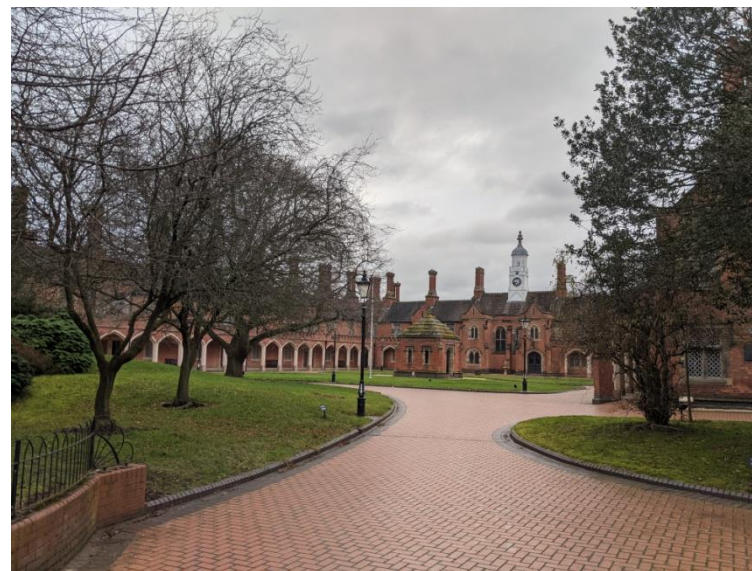
Figure 14: The Nicholas Chamberlaine Almshouses – Listed Grade historic buildings. A focal point of the town
