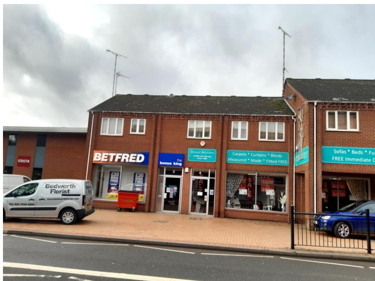
Figure 2: Modern Development on Leicester Road
