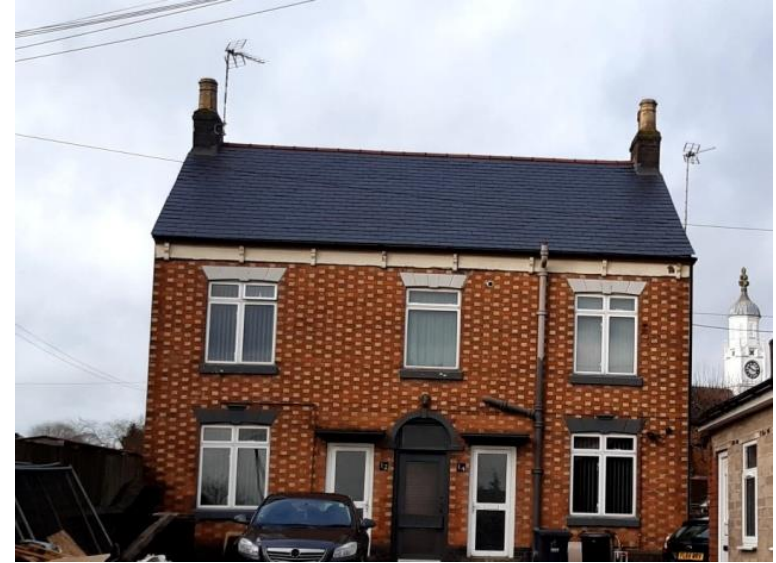
Figure 36: Distinctive Brickwork, Croxhall Street
