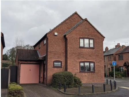
7A Chequer Street Does not contribute positively
