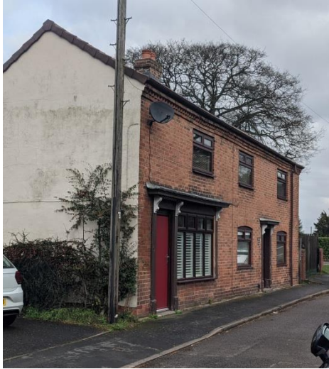
Figure 26: 10 and 10A Church Street
