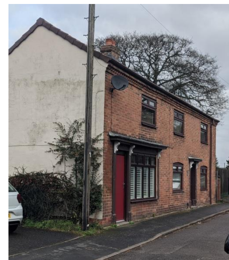
Figure 8: 10 and 10A Church Street
