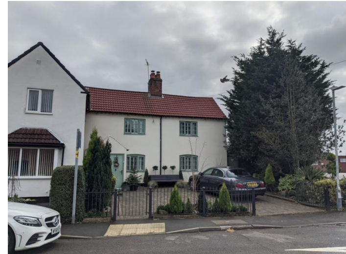
Figure 31: 30 and 31 Church Street
