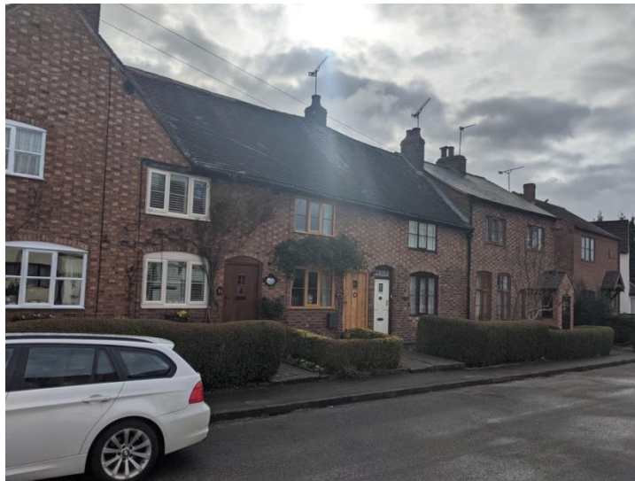
Figure 24: 25 to 28 Church Street
