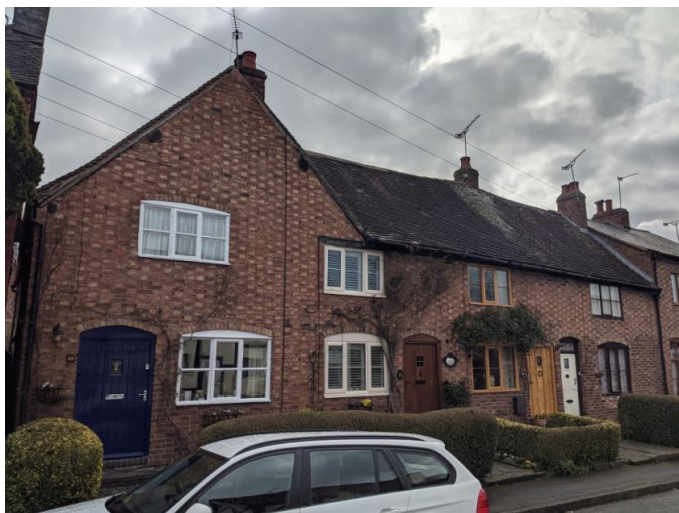
Figure 4: 25 to 28 Church Street
