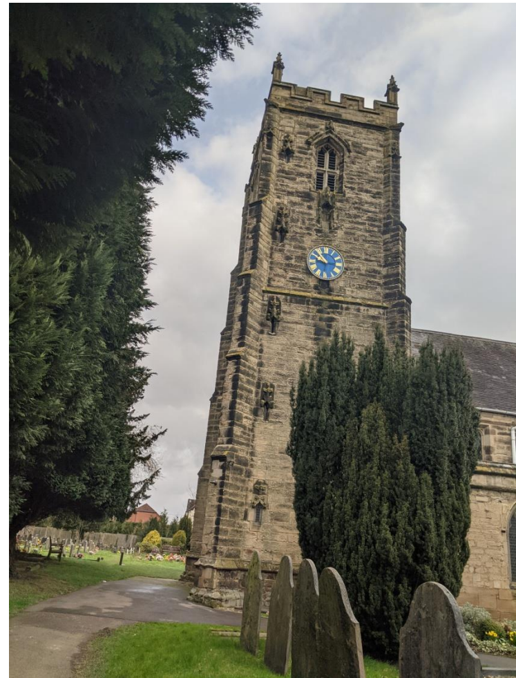
Figure 19: St. James Church from the east
