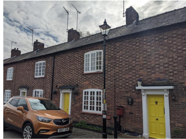
Figure 20: 3 and 4 Church Street
