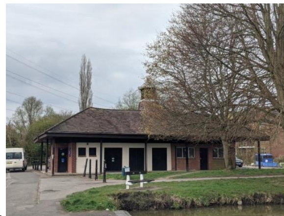
Figure 25: Central Services Building
