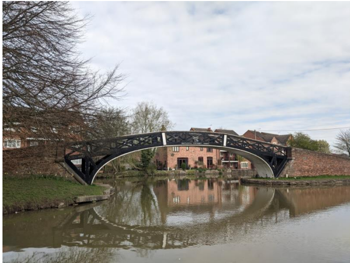
Figure 12: Footbridge over the Coventry and Oxford Canals
