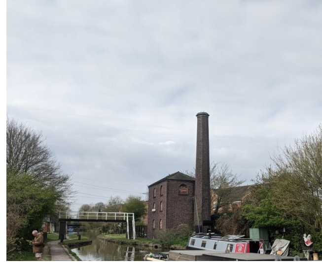
Figure 16: Northern Bank of Coventry Canal
