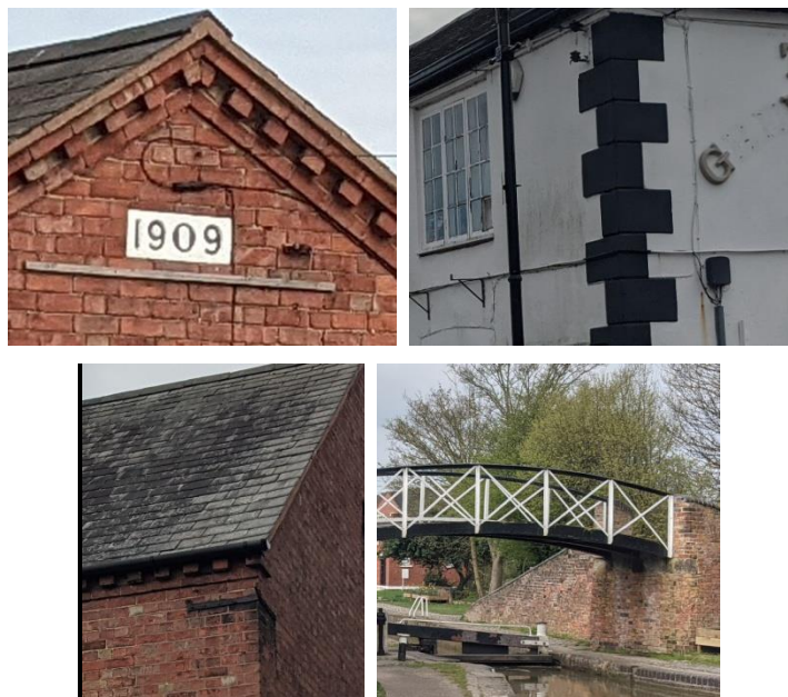
Figure 8: Decorative Details and Signage
