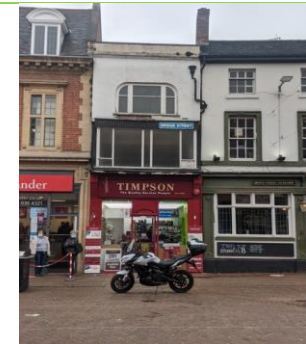
1 Bridge Street Positive
