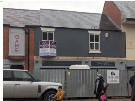
5 Queens Road Neutral
