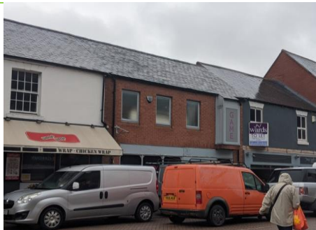
7/9 Queens Road Negative
