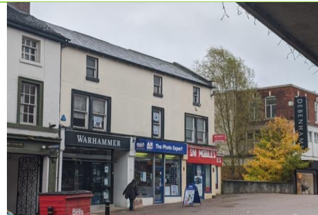
3-4 Bridge Street Positive
