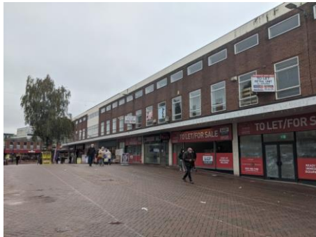
18 to 20 Bridge Street Negative
