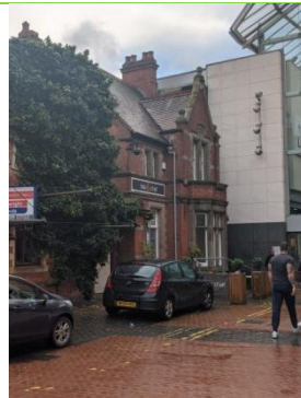
2 Chapel Street - Sycamore Tree
