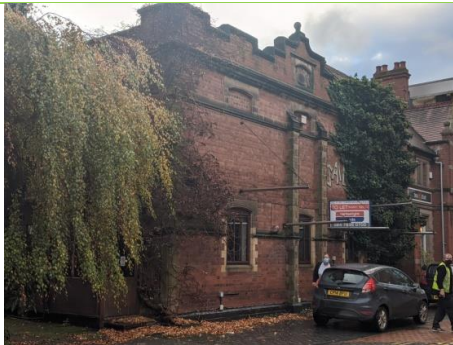
Chapel Street - Jailhouse pub
