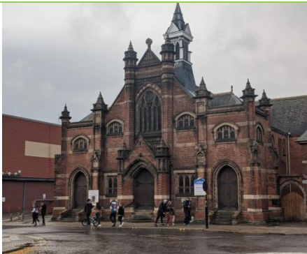
Chapel Street Nuneaton United Reformed Church Local List – Positive
