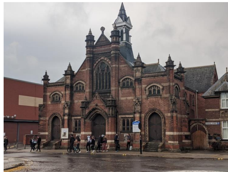
Figure 60: Chapel Street Nuneaton United Reformed Church
