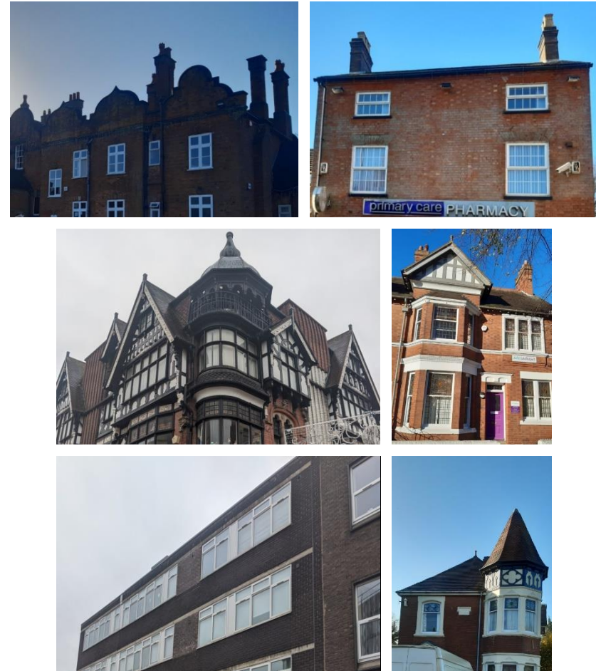
Figure 31: Roofs in the Conservation Area
