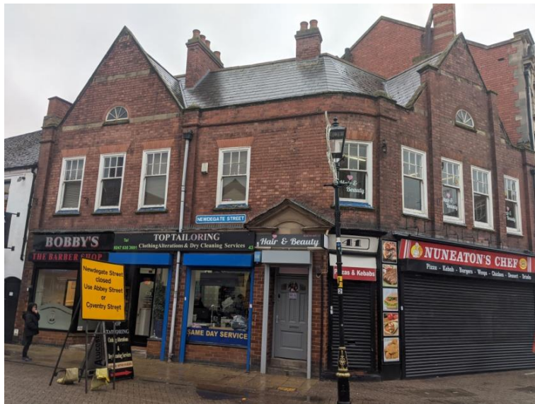
Figure 75: Signage not in sympathy with the host building
