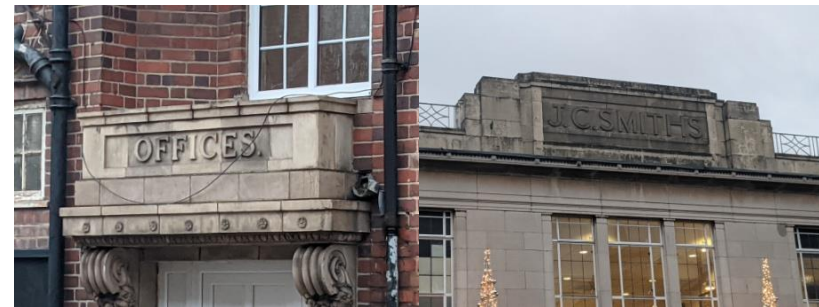
Figure 30: Decorative Details and Signage
