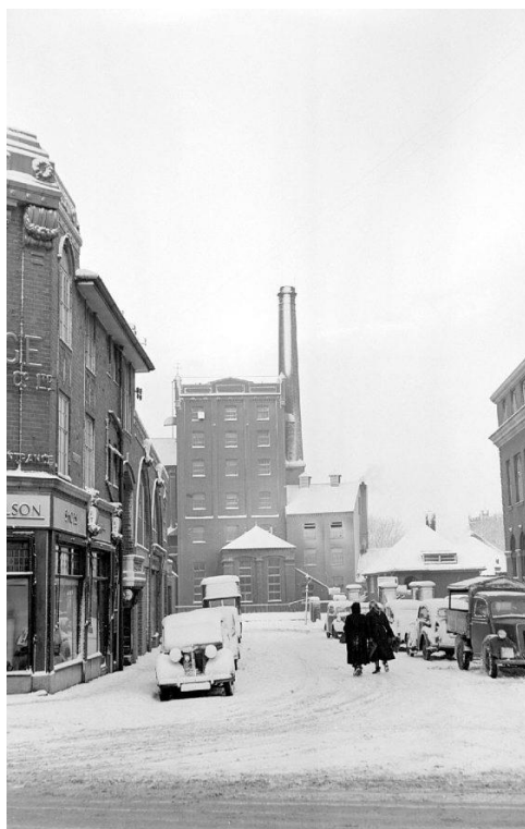
Figure 6: Nuneaton Mill, Mill Walk 11
