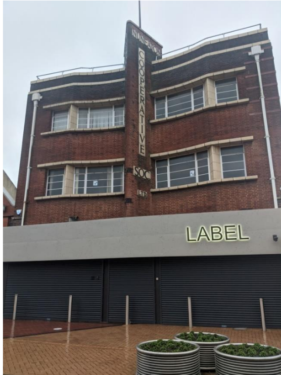
Figure 43: 23a Queens Road (Former Co-op Building)
