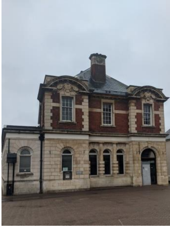
Figure 22: Former bank building, baroque freestyle, stone and brick materials, corner Newdegate Street
