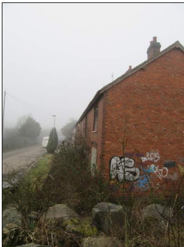
Plate 34: Detail of workers housing associated with the former Judkins Quarry Site (Strategic site HSG11).
