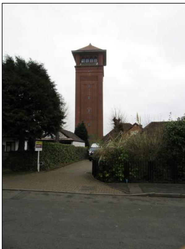
Plate 51: Detail of the Water Tower (Grade II Listed Building, NHLE: 1116416)
