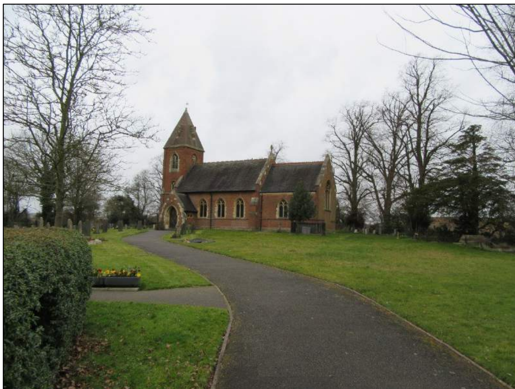
Plate 2: View from south along the main approach towards the Church of St James (NHLE: 1185771)
