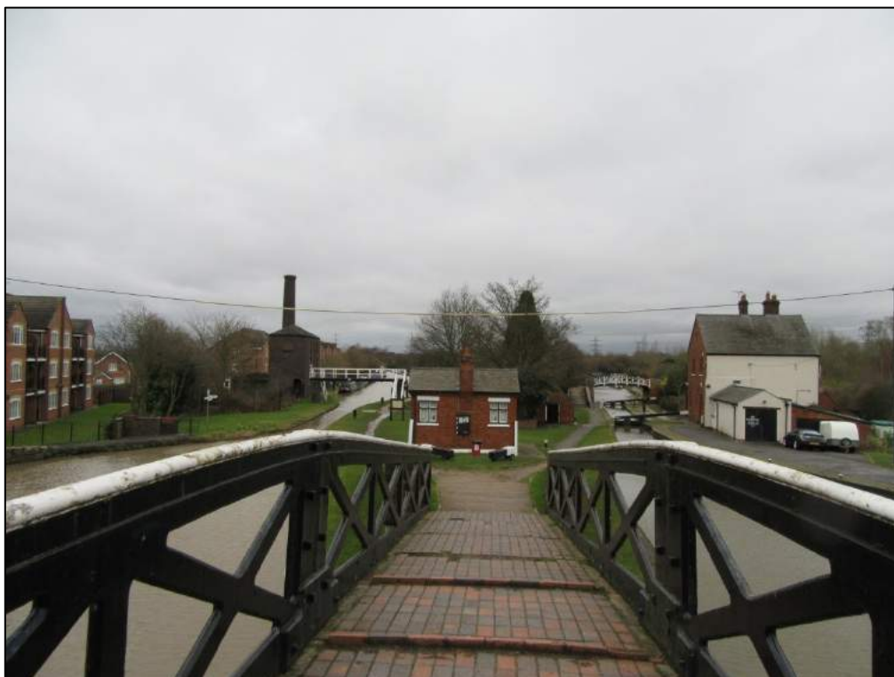
Plate 48: General view from bridge in Hawkesbury Conservation Area.
