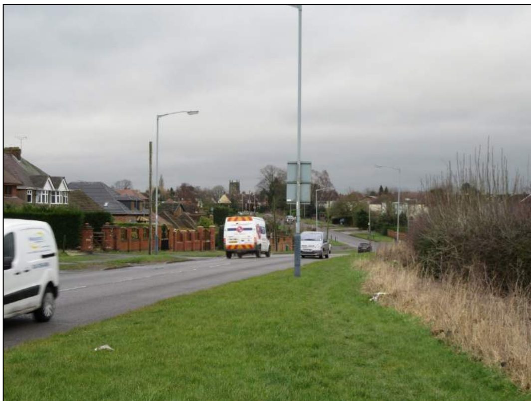
Plate 29: View from strategic site HSG8 towards Bulkington and the Church of St James (NHLE: 1365054).
