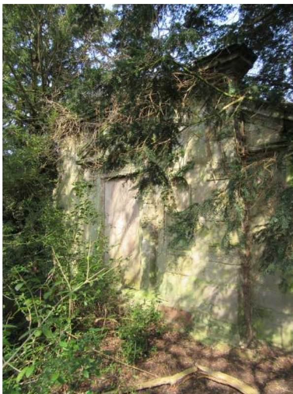
Plate 8: Detail of Arbury Hall Tea House (NHLE: 1299615)
