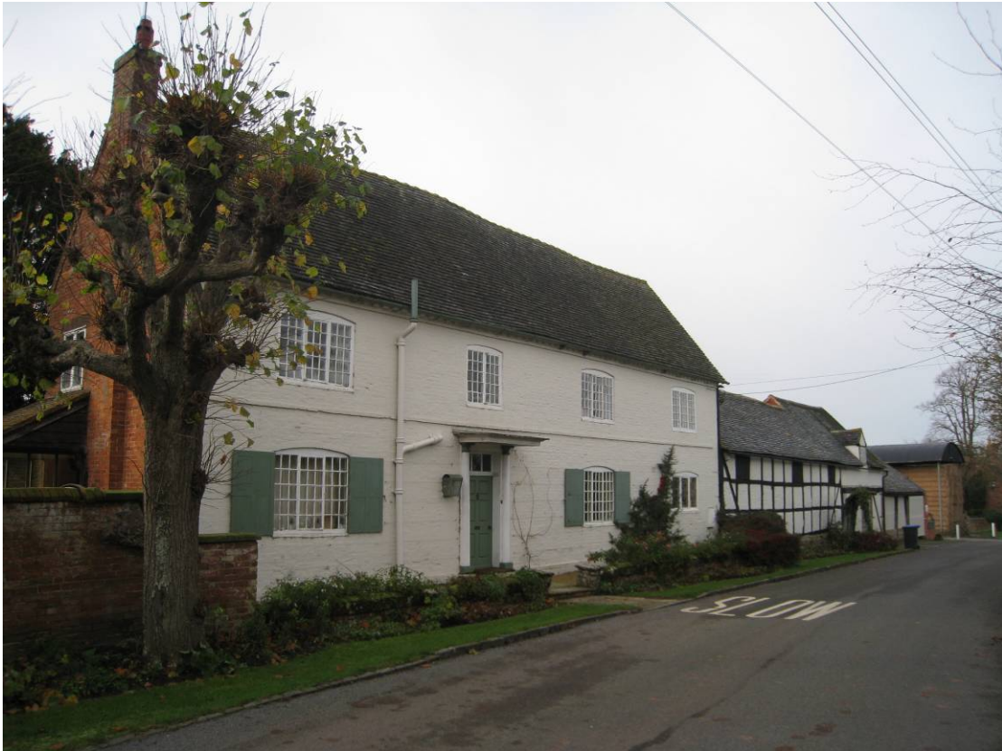
(Figure 56) Walcot Manor Farm. The 19th century re-facing may conceal an earlier timber framed building.
