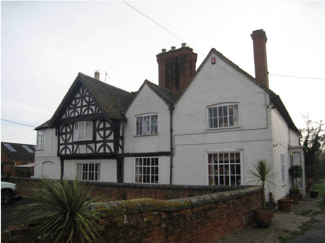
(Figure 57) Manor Farm, Upton. The farmhouse dates from the late 16th or early 17th century. The detachment of the house from surrounding working buildings may be related to the status of its builders.
