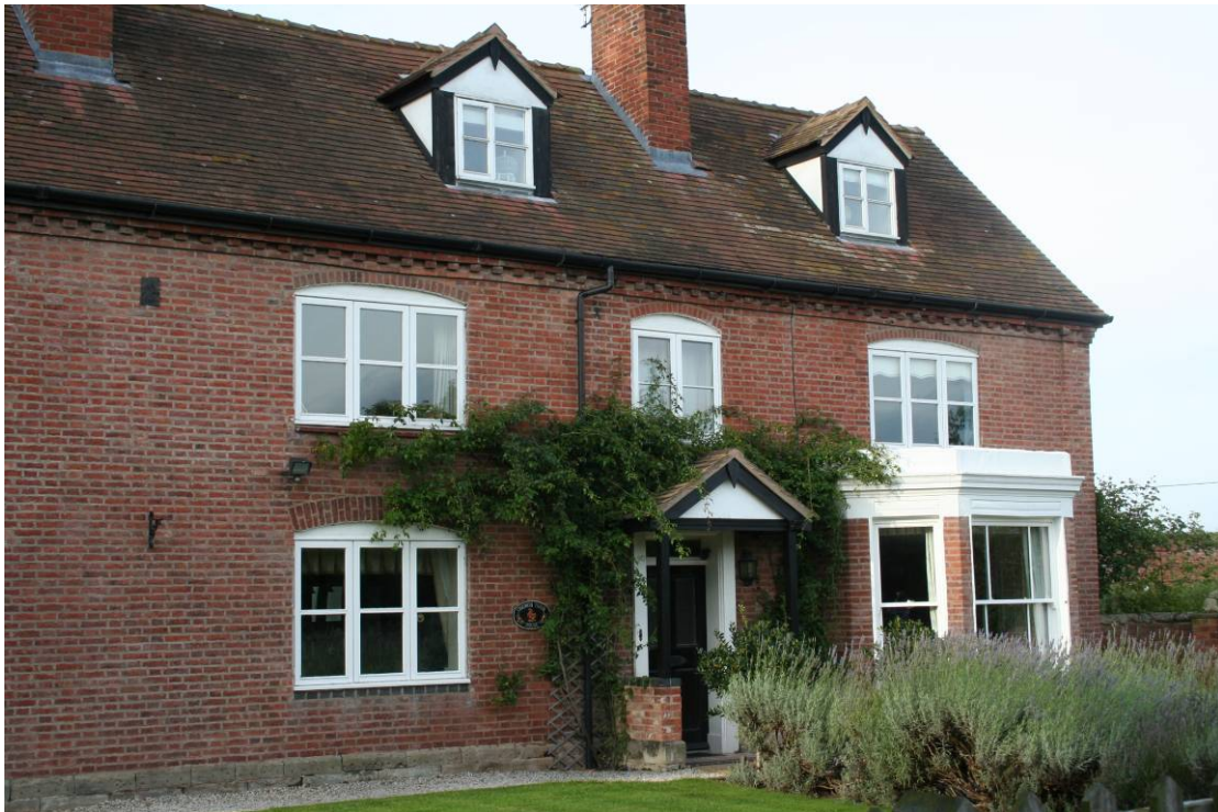
(Figure 24) Church Farm (Old Milverton, Warwick), using listed building data has under represented the extent of early fabric (i.e. pre 19th century) surviving in historic farmsteads. This farmhouse displays 18th century brick re-facing with a Flemish bound. The 18th century re-facing may conceal an earlier timber framed building. Despite this the building is not listed.
